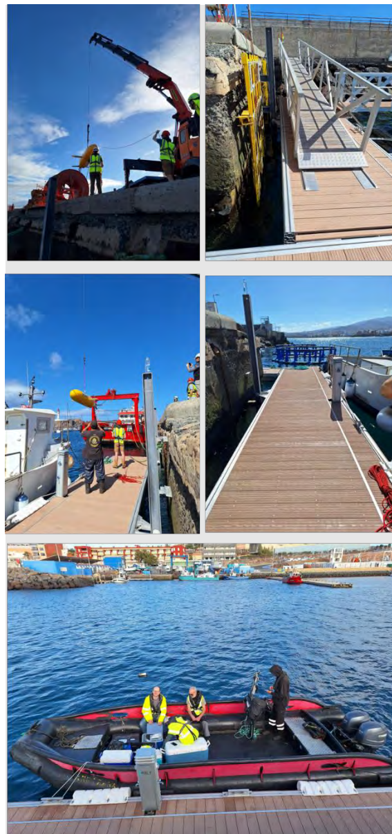
Figure 3.2. Work at Taliarte harbour.
